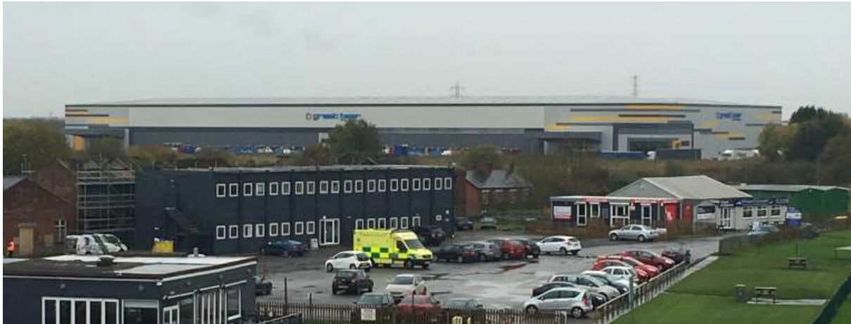
Photograph of Culina warehouse taken from the Control Tower at Barton Aerodrome
